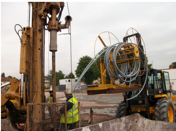
Installing Ground Source Loop in 100m deep Borehole
