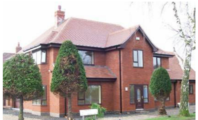
A residential property where we have installed 5 test borehole collector loops to varying depths for a ongoing long term data collection programme
