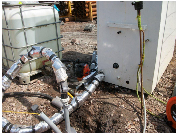
Undertaking a Thermal Response Test (TRT)
