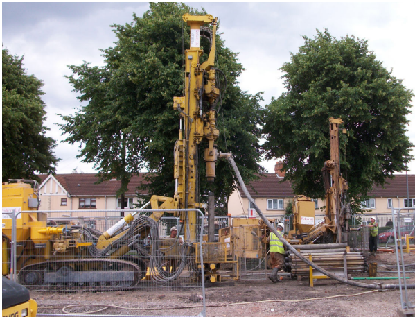
Installing Borehole Collector Loops for New School
