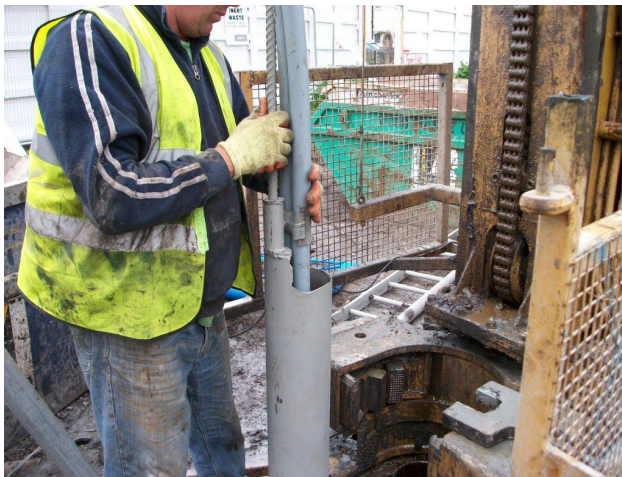
Installing a Collector Loop in a Borehole
